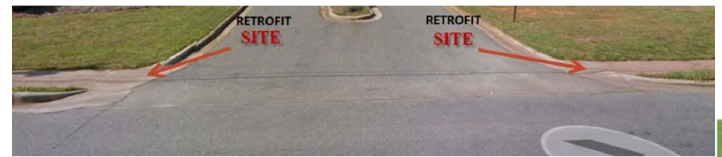
US 70 at CLAREMONT PARK ENTRANCE
