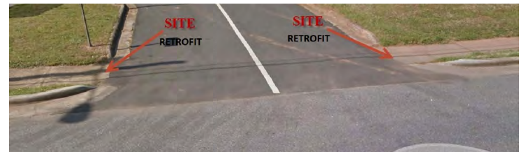
US 70 at SCHOOL ENTRANCE
